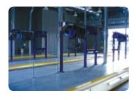
The finished pit is now complete with state of the art Diagnostic Equipment, Jacking Systems, Lighting, Ventilation & Water Recycling.
