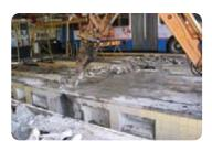
First steps are to break the existing concrete on floor level to accommodate the brake and suspension testers.
