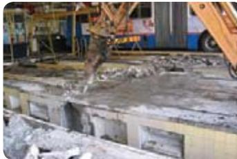
First steps are to break the existing concrete on floor level to accommodate the brake and suspension testers.
