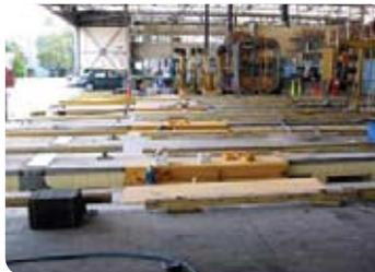
Layout steel work to carry the jacking system and locate jack runs on pit wall and secure to wall or structure.
