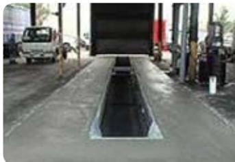
Lay formwork on pit floor for concreting, pour concrete to form the new finished floor. Weld in top deck steel work and paint pit in two pack epoxy. Pit jacks plumbed to external power
